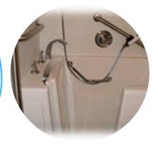
All valves and control mechanisms should be operated by a lever, and all flow valves should turn to full flow capacity within a quarter-rotation of that lever.
