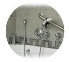
One is through an ADA compliant anti-scald shower valve that is plumbed to a separate handheld shower with the filler system plumbed through its own thermostatic valve.
