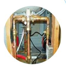
By far the best technology is what is referred to as a "Type T" anti-scald valve. These mixing valves are true "True" valves. That is what the "T" stands for.
